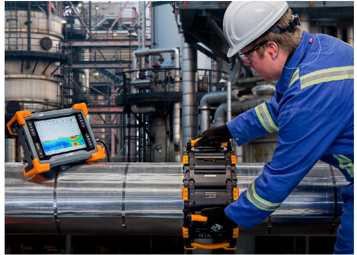
Figure 4: Lyft PECA pipeline CUI.
